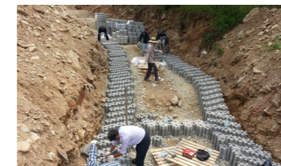
It can be installed with human labor only in the areas inaccessible by equipment
