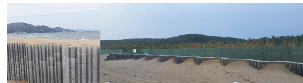
Can be installed without foundation prepping work so that overall construction time can be reduced
