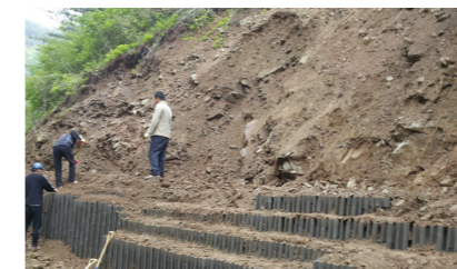
Can be installed without foundation prepping work so that overall construction time can be reduced
