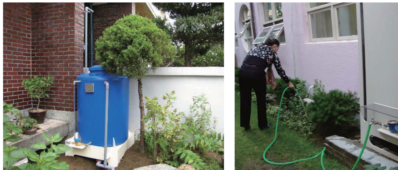
Collects rainwater to be used for various purposes such as flower bed and others
